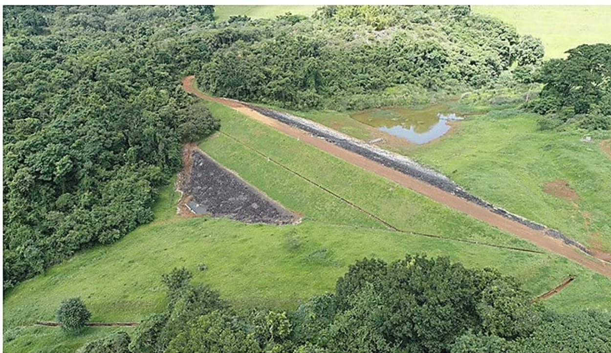
Figure 2 – photo of Dam D. Source: https://cbmm.com/en/our-company/our-dams
