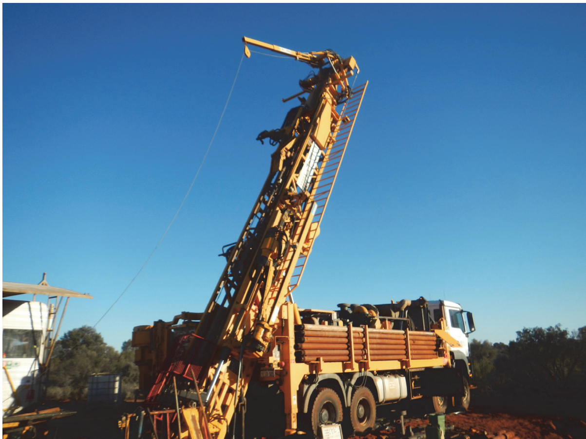
Figure 1 – drill rig at Desert Dragon Central
