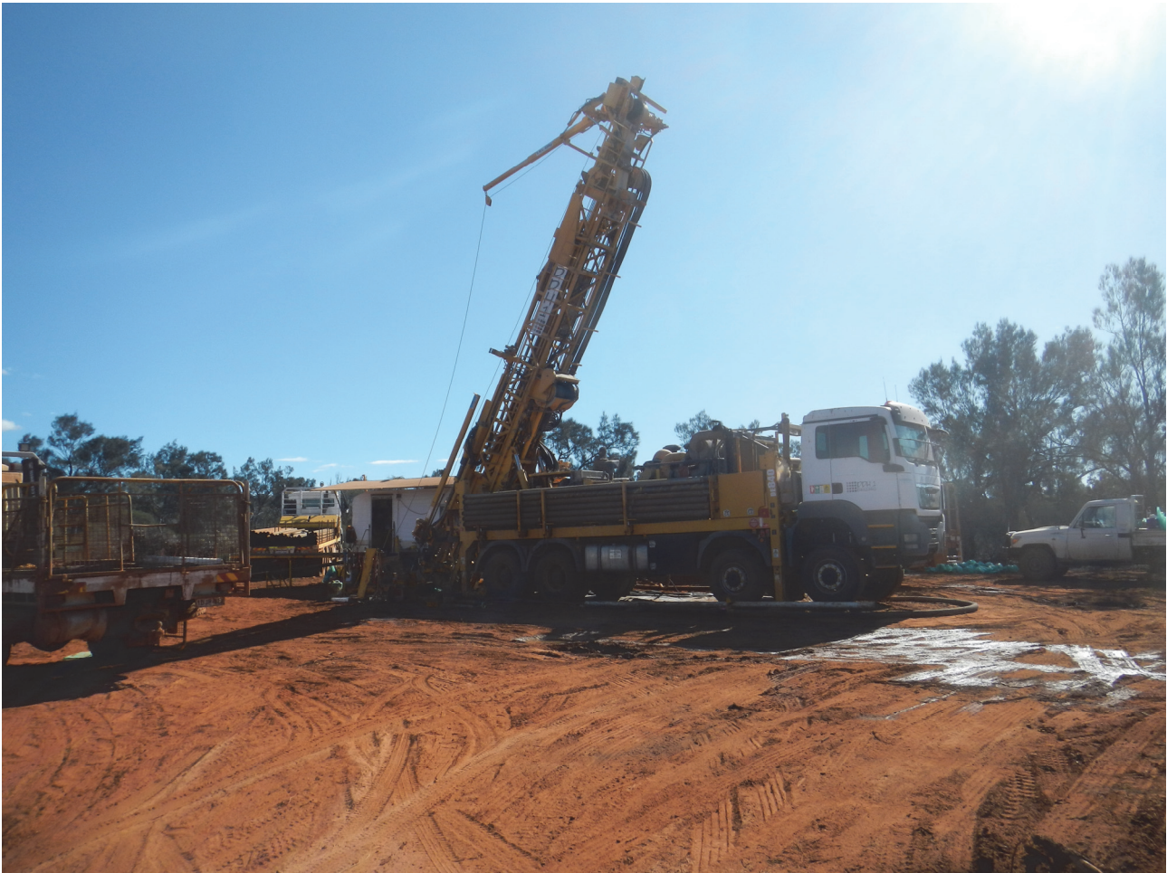
Figure 1 – the drill rig at Cambridge
