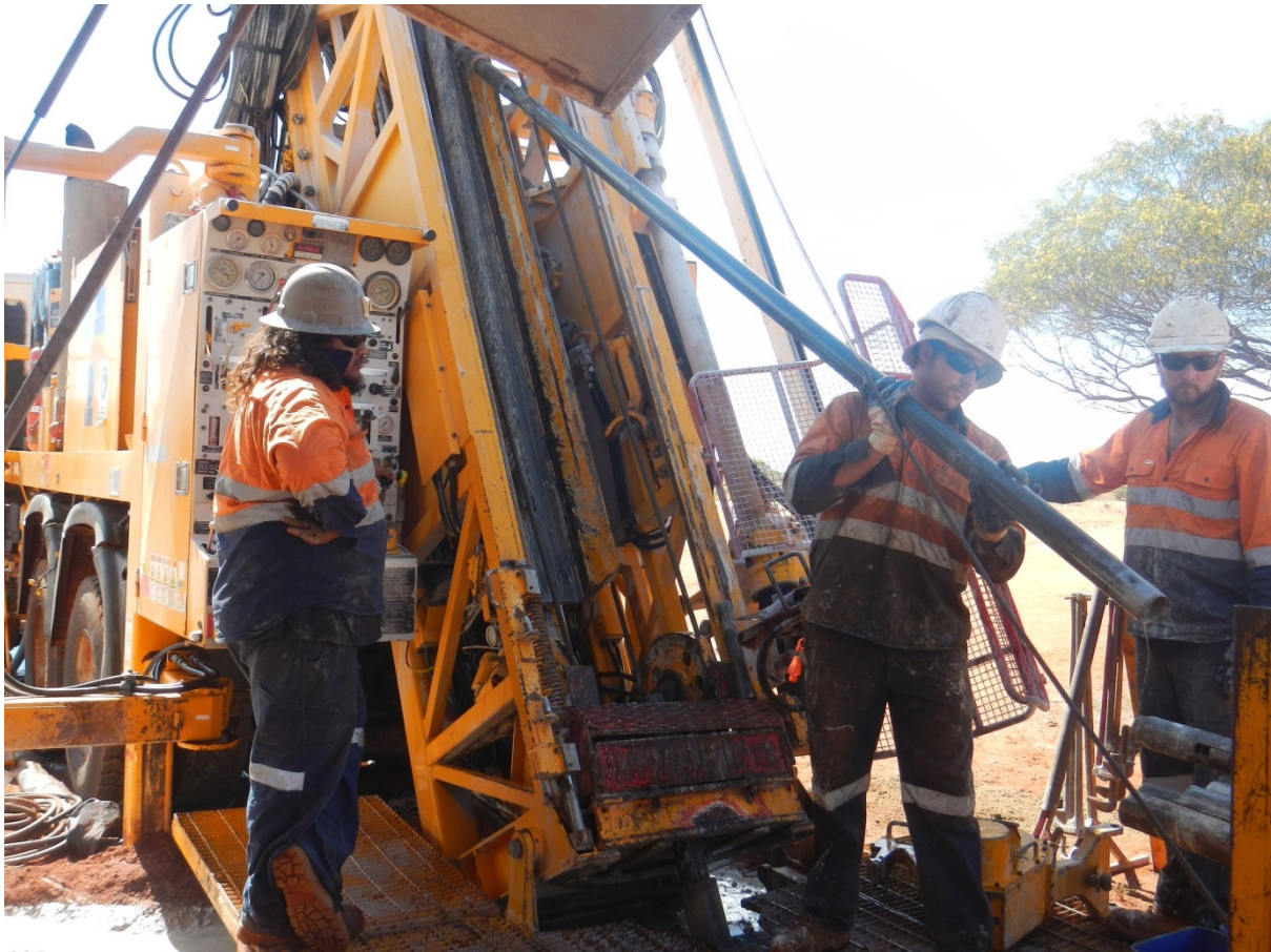
Drilling of EM conductors at Mt Alexander
