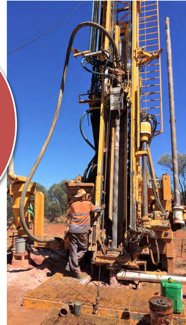
On right: Diamond drilling at Mt Alexander
